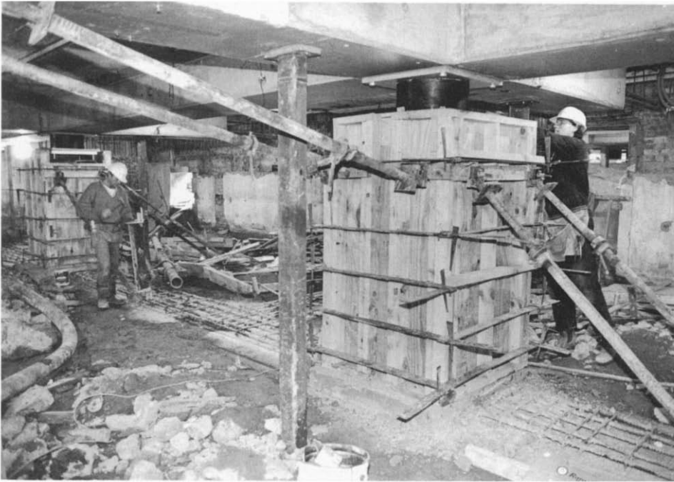
Fig. 4. Lead-rubber bearings being retrofitted under New Zealand Parliament Building, 1993.
